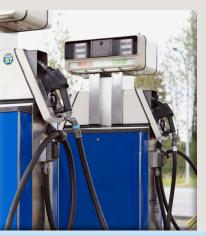
Turn off power to electrical systems such as pumps, turbines, dispensers, ATG consoles, emergency shutoff panel boxes, etc. Check fuel levels in each tank for later comparison.
