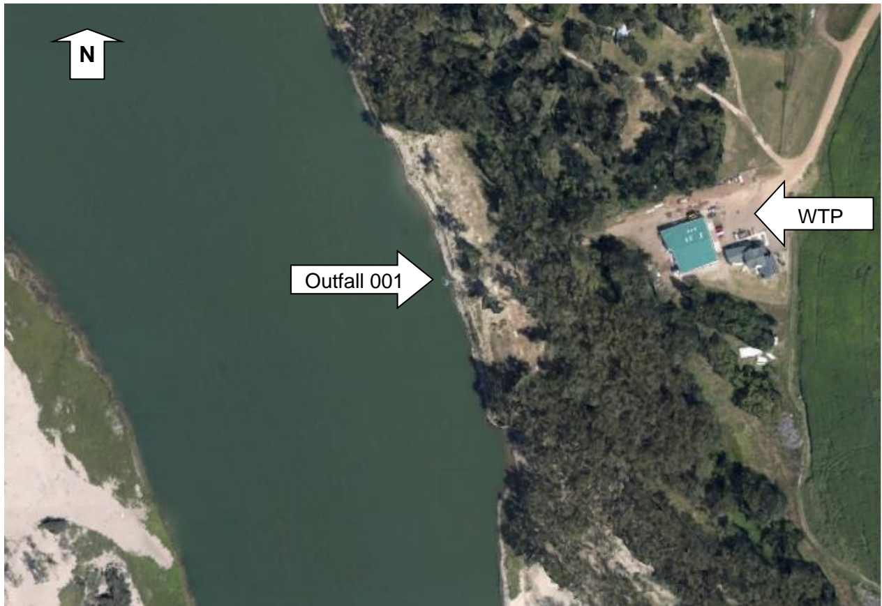
Figure 1 – Aerial photograph of South Central Regional Water District - North Burleigh Water Treatment Plant (Google Earth 5/30/2017). Image does not show new sludge pond.
