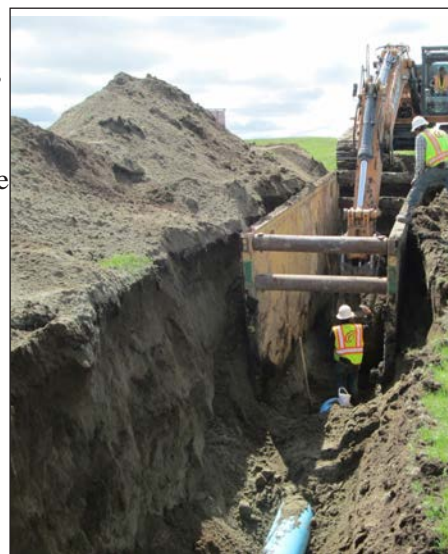
Trenching pipe to further extend Southwest Water's distribution.
