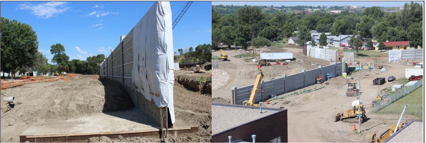
Image 1: This perspective of the floodwalls being built to protect the Minot Water Treatment Plant shows how much more concrete goes into the belowground foundation for the 14-15 foot tall floodwalls.
