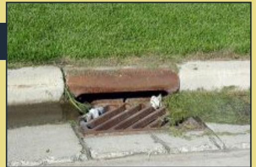
Stormwater Inlet (Courtesy of http://www.grandforksgov.com/government/engineering/land-development/stormwater-information )
