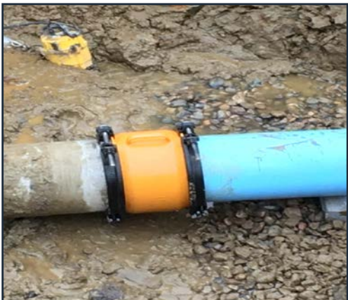
Connection of Rugby's new and old water main (Courtesy of Interstate Engineering)
