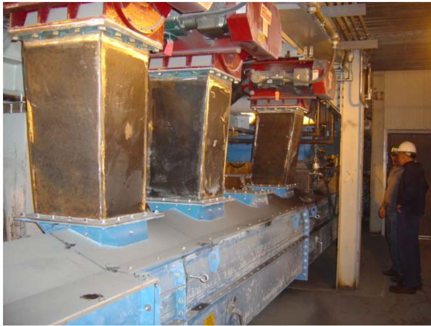
Figure 1-8: Dried Coal is Discharged through Three Rotating Coal Feeders
