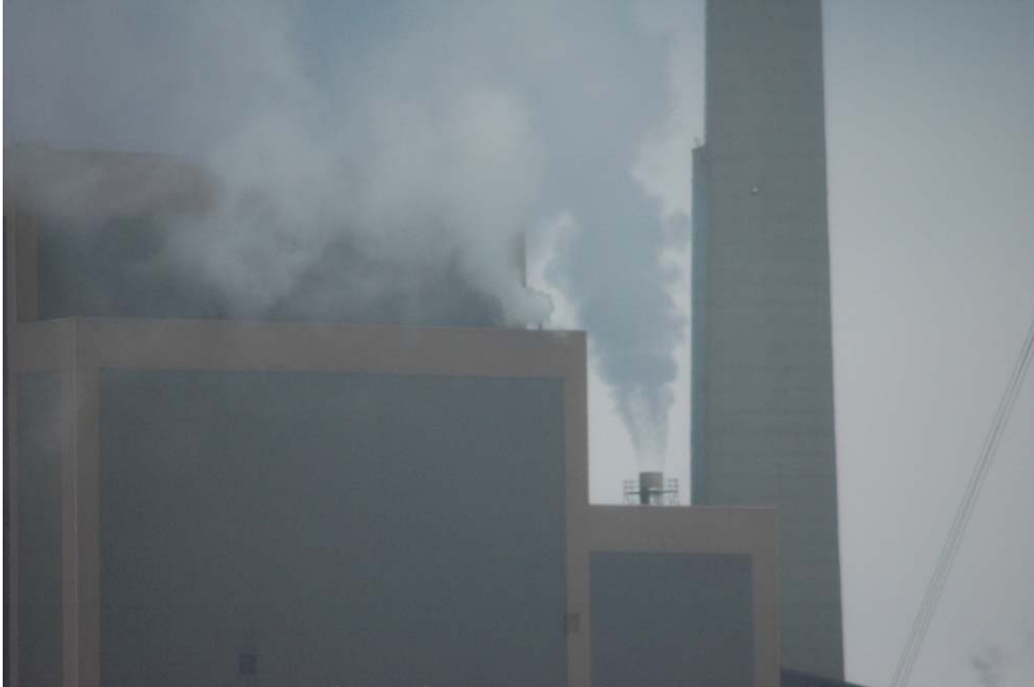
Figure 1-9: Clean Moist Air Stream Leaving Dust Collector is Discharged into the Atmosphere
