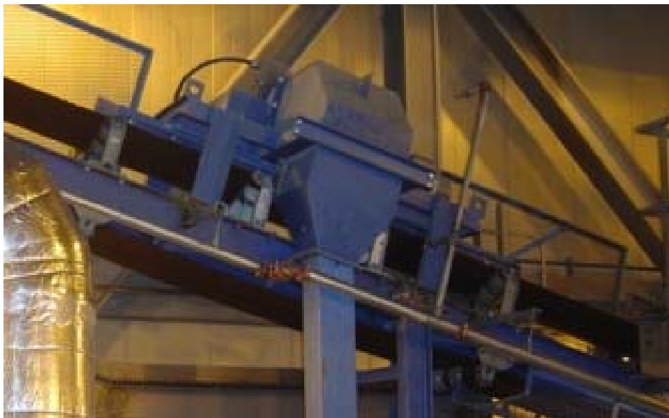
Figure 1-11: Automatic Coal Analyzer: Feed Conveyor
