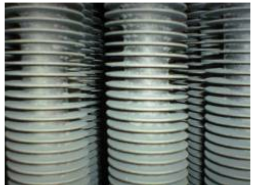
The State of the Heating Tubes (After 2 years of operation)
