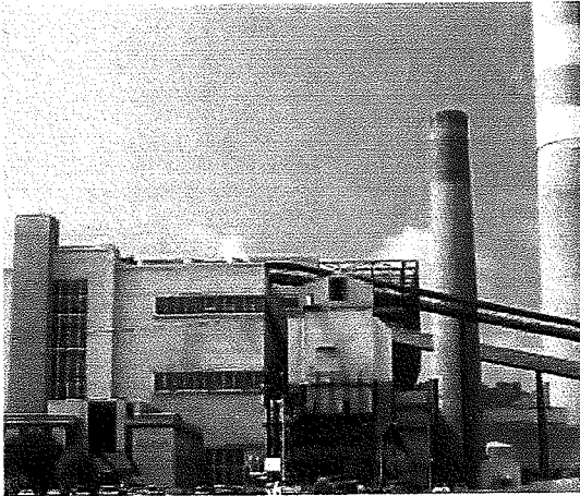
Advatech is currently designing a single-module DCFS FGD system for Alabama Power's 1,151 MWe Plant Gorgas which will achieve 98 percent SO 2 removal efficiency with ultra-high reliability.
