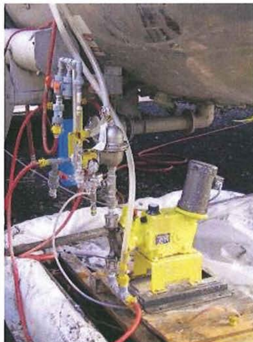
Figure 2-4 Dilution/Booster Pumps at Elevation 457 Feet
