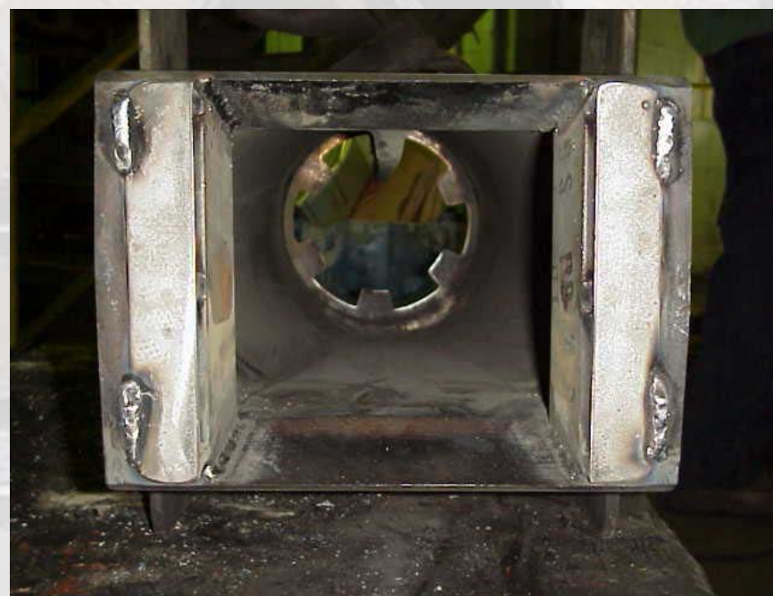
ACT Coal Pipe Inserts positioned inside existing coal pipe
