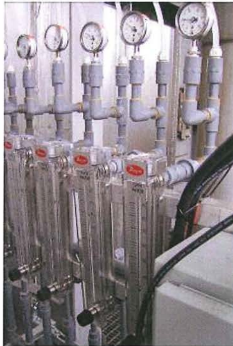
Figure 2-5 Distribution Header at Elevation 457 Feet
