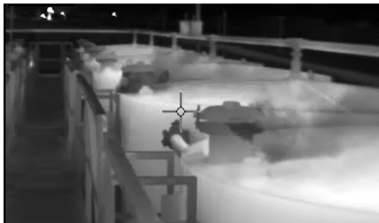
Infrared video image of thief hatch emissions.
