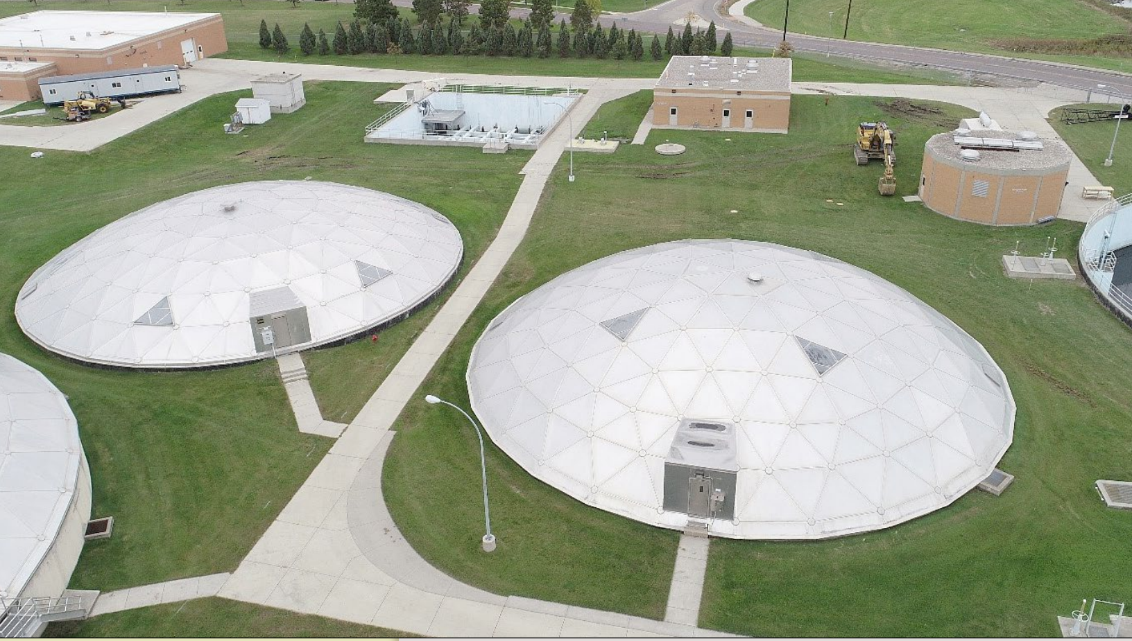
Fargo's wastewater treatment facility
