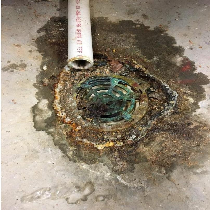
Washes away surrounding concrete, metal drains and piping. This is after 3 years.
