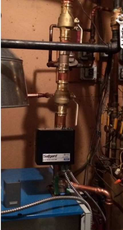
Probe Style Low Water Cutoff
