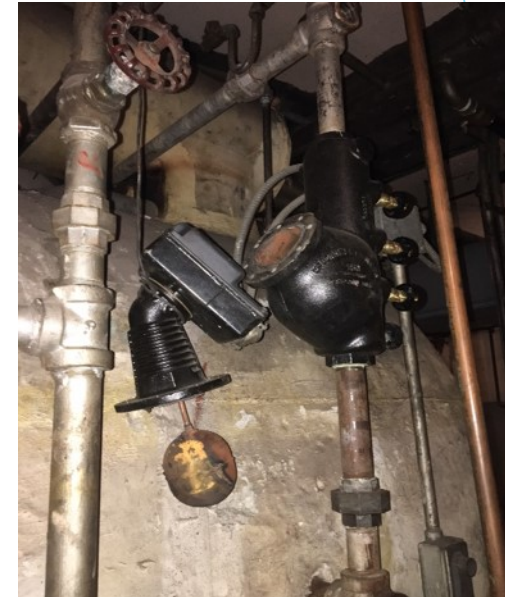
Low water cutoff float bowls split open to see inside bowl and check for scale/mud. Check condition of float.
