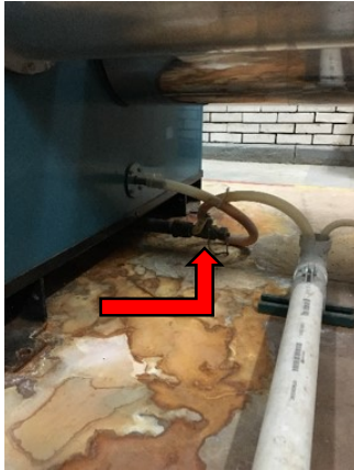
Condensate Loop Seal at Back of Boiler
