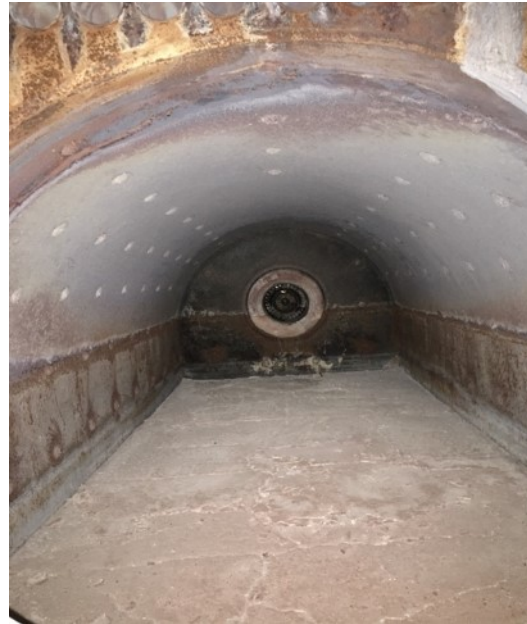
Firebox - no distortion of metal, no leaking stays, refractory/firebrick in good condition.
