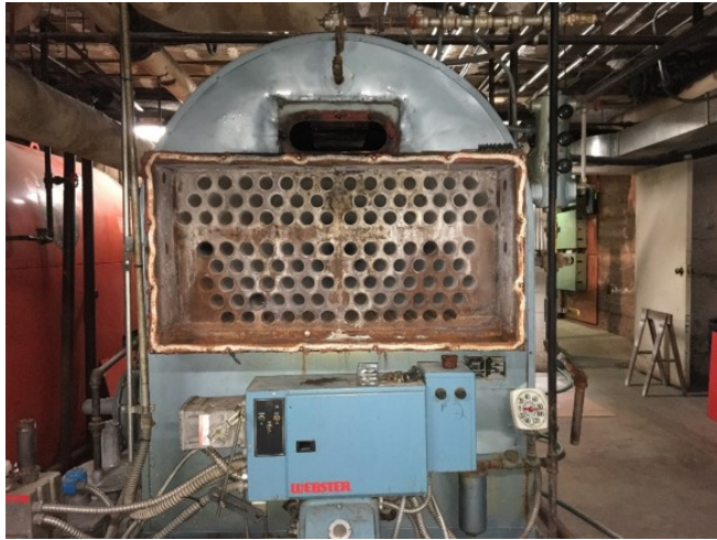
Fire sides of tubes brushed clean. Check for leaking tubes/tube rolls. Condition of tube sheet.
