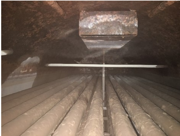
Water side of fire tubes and shell of boiler. Check for scale and pitting on tubes and shell. Distortion of any parts.
