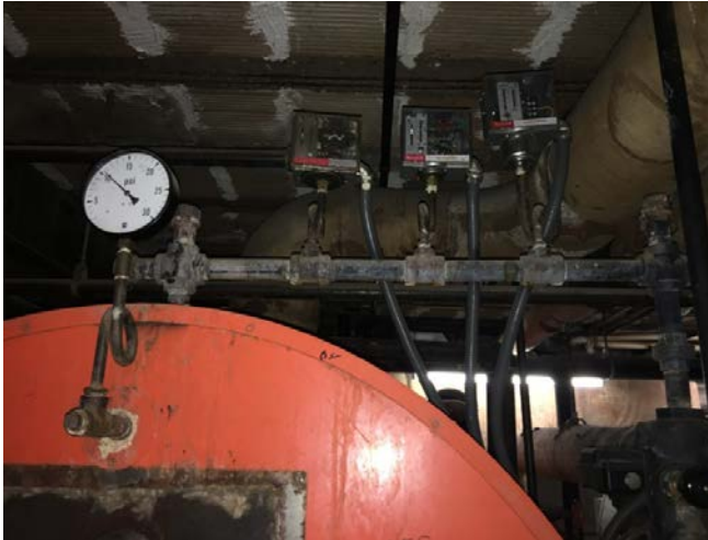
This boiler shown above has three pressure controls - operating, high limit and the third could be for modulation or high/low fire.
