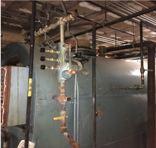
The MM 157 low water cutoff shown above has a gauge glass and gauge cocks installed.
