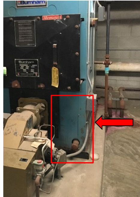
Check stays for thinning. Check shell plate distortion, pitting and scale. Check bottom of mud legs for corrosion and pitting.
