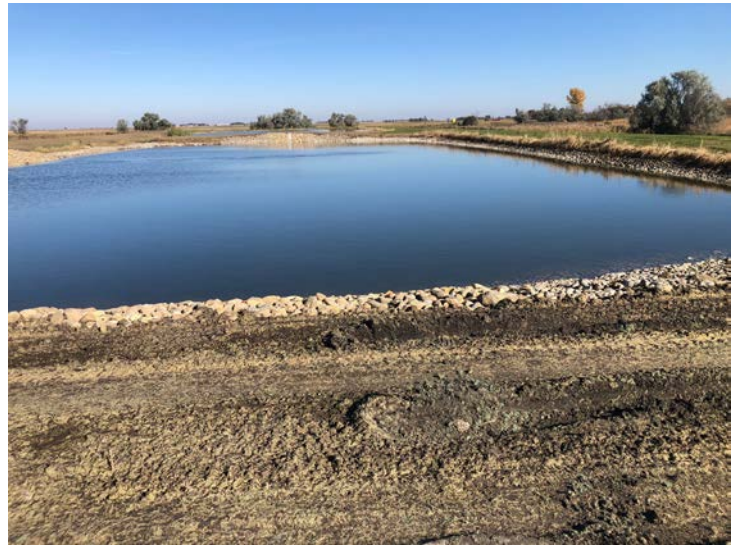
Pictured is a wastewater stabilization lagoon located in Rutland, N.D. Facultative pond systems, such as this, use natural processes to treat wastewater. Credit: Shawn Martin
