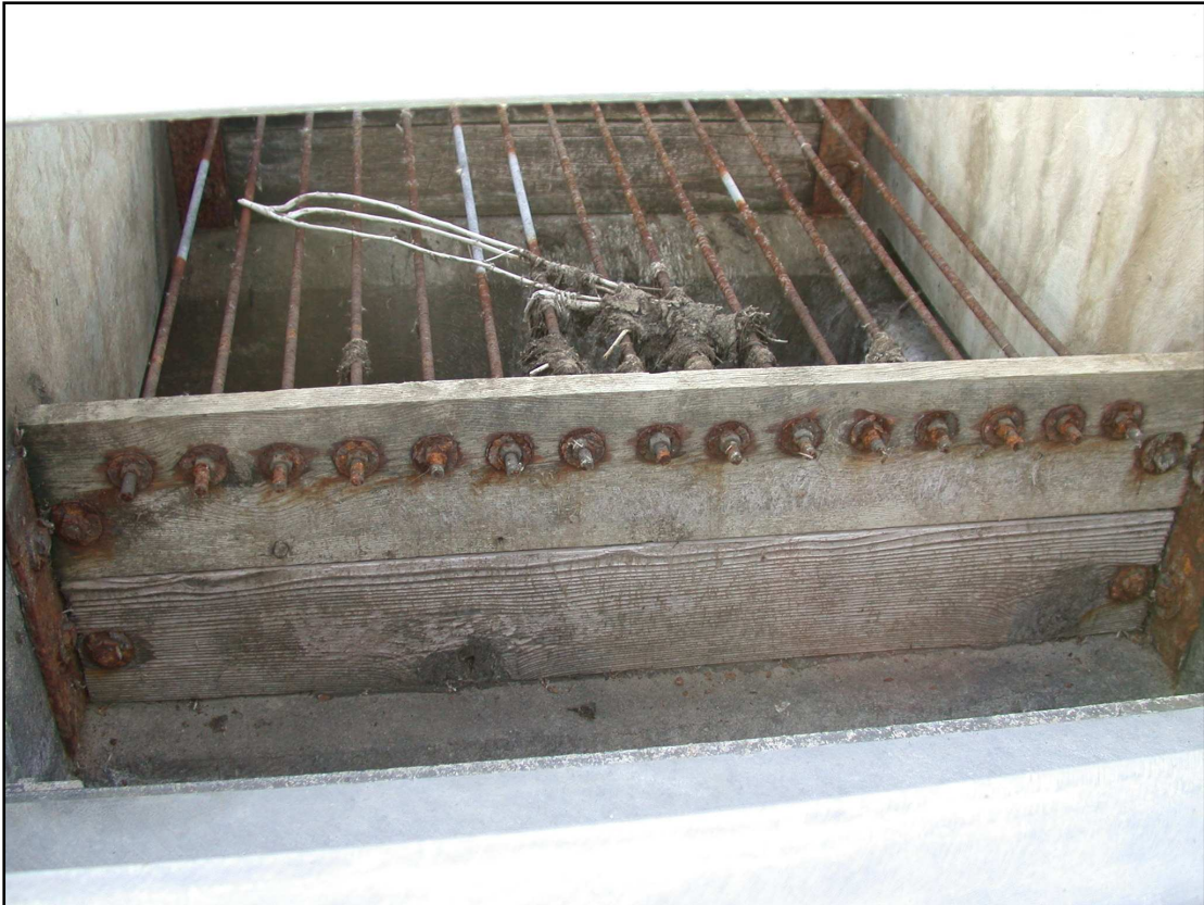
Redwood flashboards installed in 1980 to raise the effective outfall elevation of McDowell Dam from 1723.5 to 1724.56.
